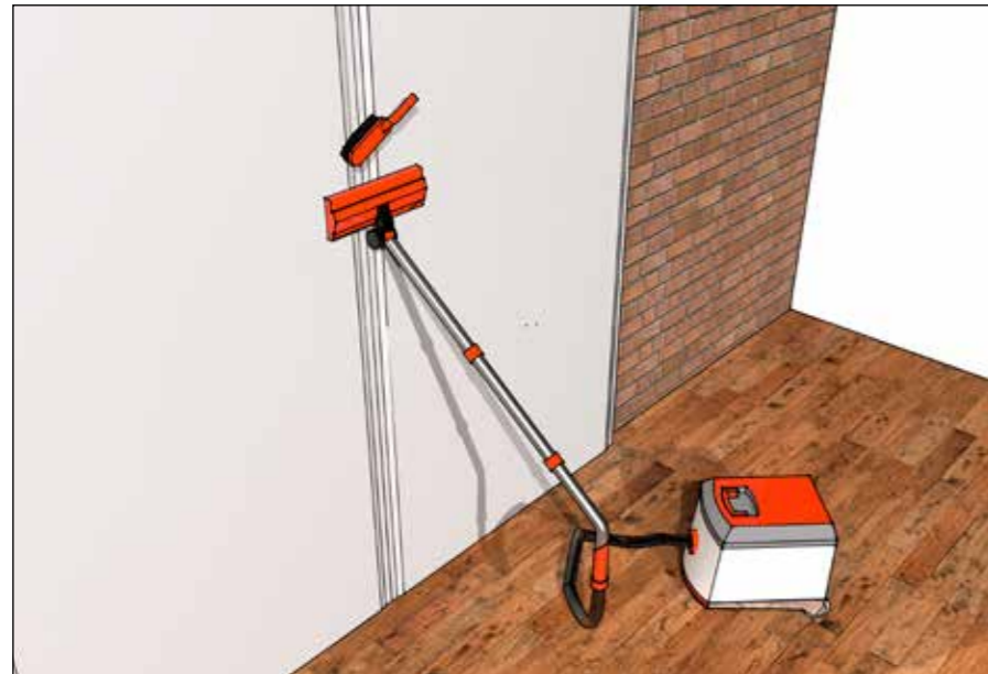
Fig. 7 Preparing Spacetherm Wallboard surface for jointing
