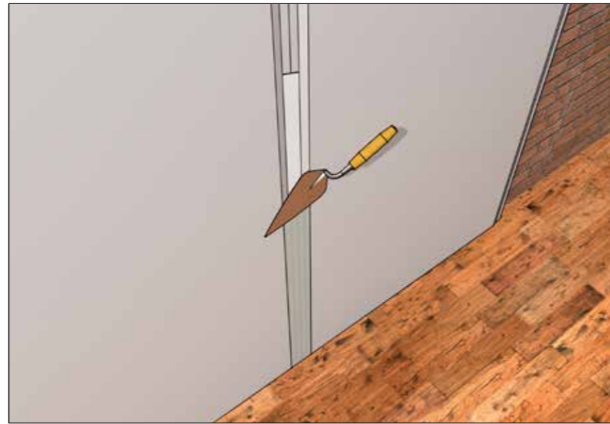
Fig. 8 Taping and Filling Joints in Spacetherm Directfix / Spacetherm A2 Directfix
